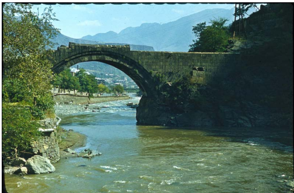
Debed river and Sanahin bridge
